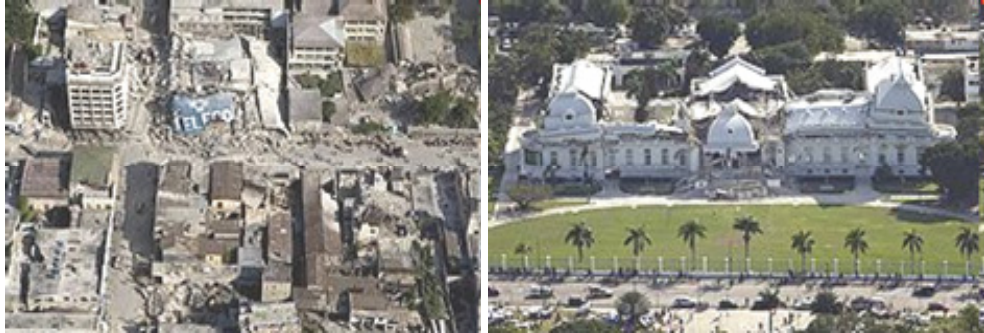
Fig. 2. Sudden geological event. Earthquake Haiti, registered on January 12, 2010 at 16:53:09 local time (21:53:09 UTC) with epicenter at 15 km from Port au Prince, Haiti's capital. Views of National Palace and collapsed buildings in downtown Port au Prince.
